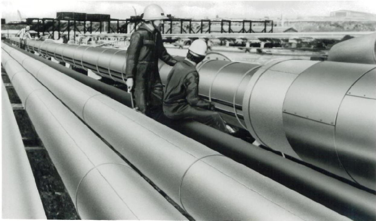
Pipelines provide a simple means of transporting materials, liquids, powders, and gasses over sometimes relatively long distances, both efficiently and inexpensively. When thermal insulation alone is not sufficient, then the pipeline needs heating.
